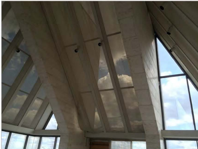
Penthouse Interior Detail
