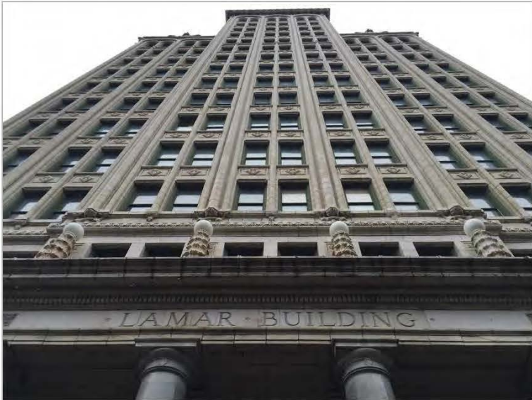
"Lamar Building" Carved Entablature
